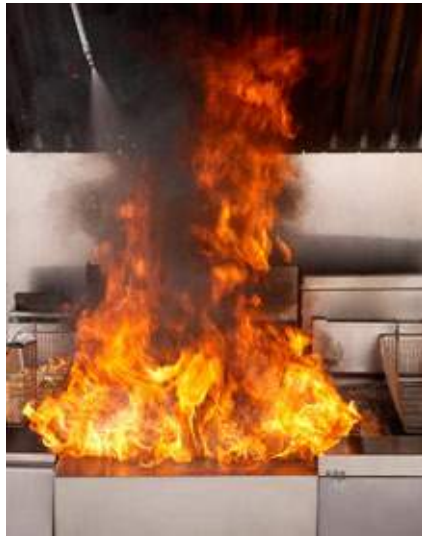
SYSTEM ACTIVATED Time = 15 seconds
